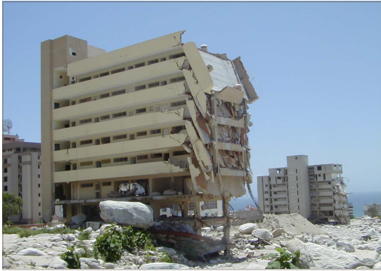
USGS OFR-01-0144 photo of Caraballeda, debris flow of "an estimated 1.8 million tons." Thousands died as their homes and apartment buildings were destroyed.
